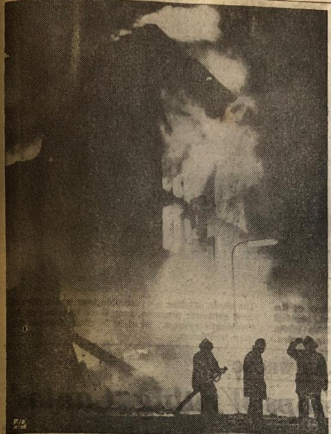
TERRE HAUTE FIRE —Firemen attempt to control flames in Terre Haute, Indiana's business district. At least eight stores were destroyed by the blaze which was pushed along by strong winds. (AP photo)
